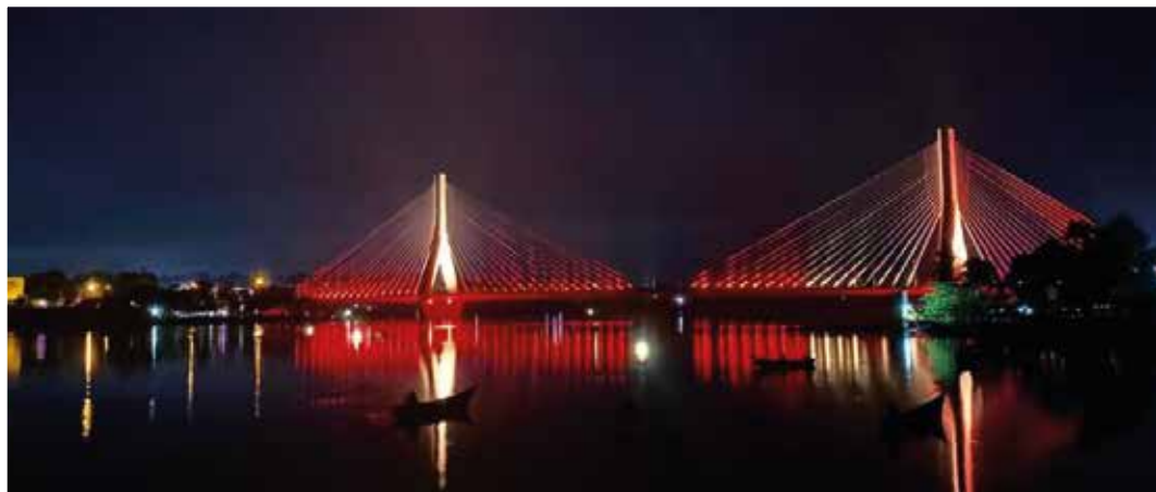
The New Nile Bridge. The Road Fund finances maintenance of all bridges.
