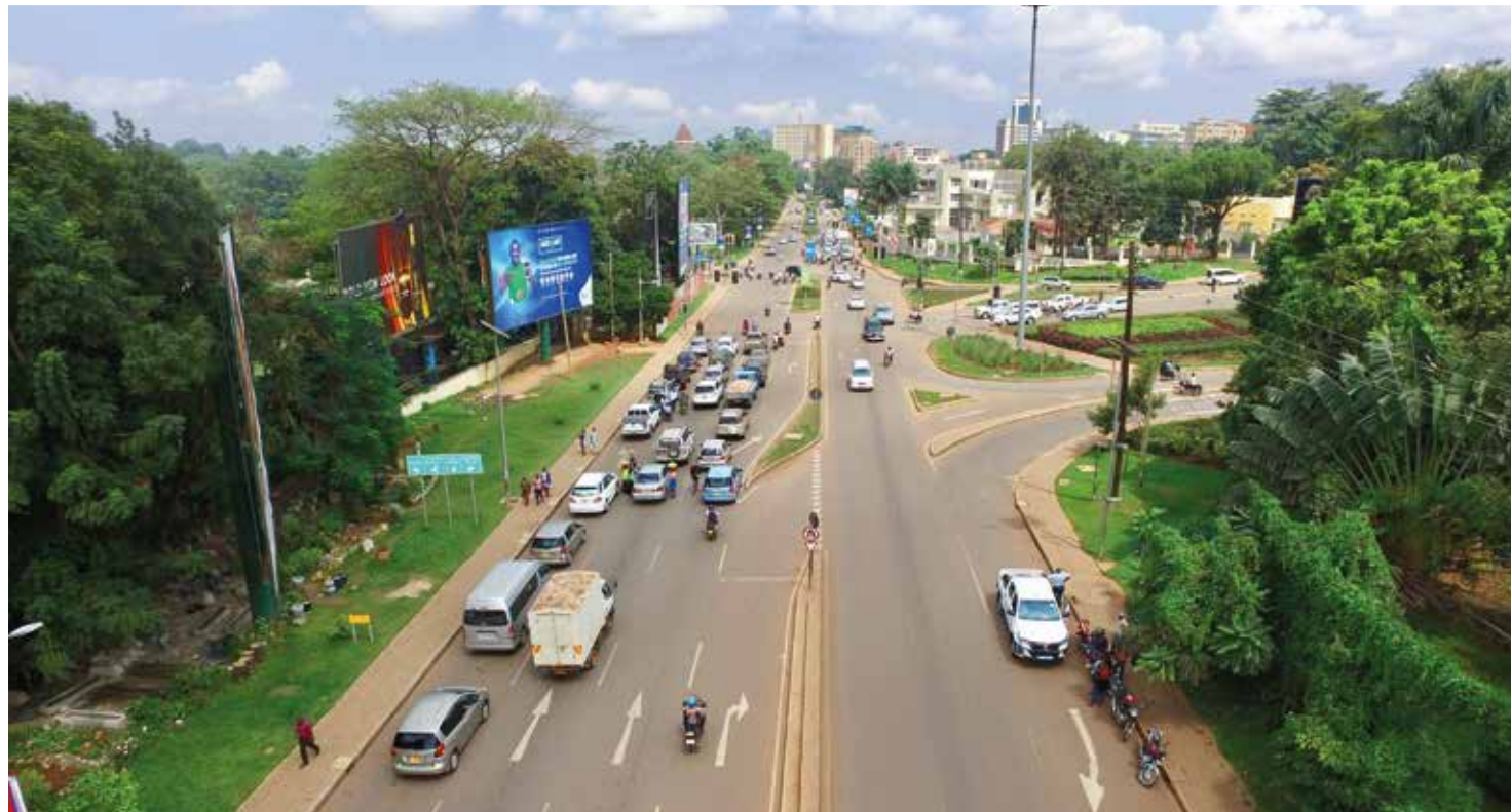
Road Fund finances maintenance of Kampala City roads, Aerial View for Yusuf Lule Road Traffic Lights Junction.
